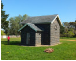
Former Bannockburn Lock Up
