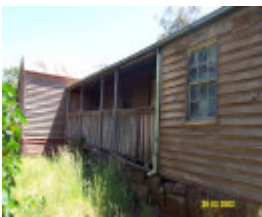
23526 Hillview Nareen verandah 1965
