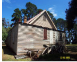
23541 Strathkellar Mechanics Institute 1907
