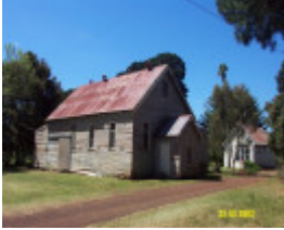
23541 Strathkellar Mechanics Institute 1904
