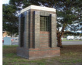
Underground toilet_West Melbourne_May 2007_brick ventilator
