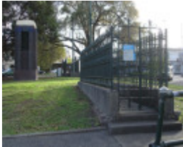
Underground toilet_West Melbourne_May 2007_general view
