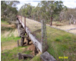
23621 Railway Trestle Bridge Wannon 1336
