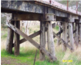
23621 Railway Trestle Bridge Wannon 1332
