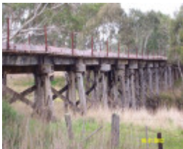
23621 Railway Trestle Bridge Wannon from W 1331
