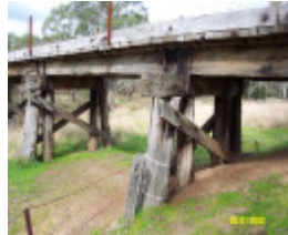
23621 Railway Trestle Bridge Wannon 1335
