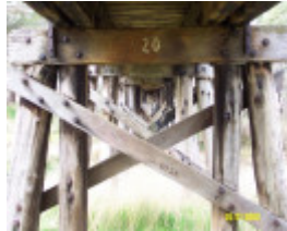
23621 Railway Trestle Bridge Wannon 1333
