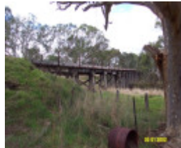
23621 Railway Trestle Bridge Wannon from W 1330
