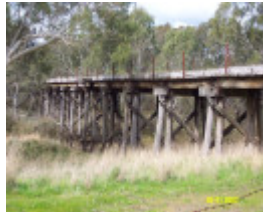
23621 Railway Trestle Bridge Wannon from E 1334
