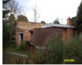
23643 Eaton Park Glenthompson east addition 1220
