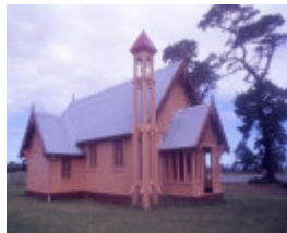
tarraville church tyers street tarraville left front she project 2004
