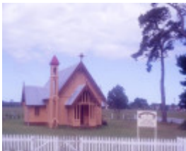
tarraville church tyers street tarraville front view she project 2004
