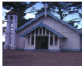
h00999 christ church tyers street tarraville front view feb1982
