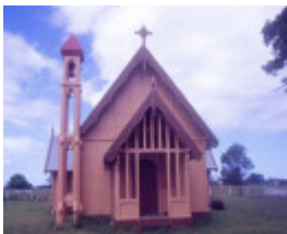
1 tarraville church tyers street tarraville close up she project 2004
