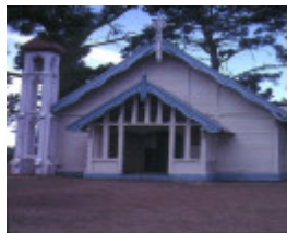
h00999 christ chuch tyers street tarraville front view feb1982
