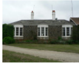
Woolbrook Homestead south elevation
