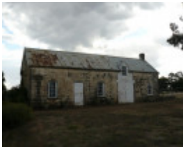
Old Stables, located north of new house.
