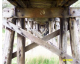
23798 Railway Trestle Bridge Wannon 1333
