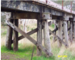
23798 Railway Trestle Bridge Wannon 1332
