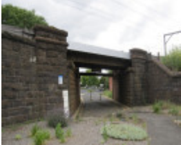
Bloomfield Road Rail Overbridge.JPG
