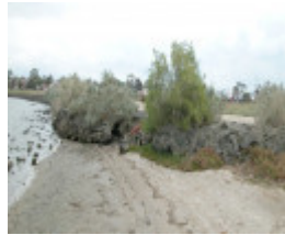
Newport Power Station Williamstown April 2003 Ash Ponds Spillway 002
