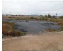
Newport Power Station Williamstown April 2003 Ash Ponds 001
