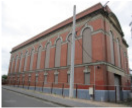
Newmarket Railway Substation.JPG
