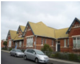
Ascot Vale PS 2608 1885/8 building
