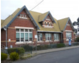
Ascot Vale PS 2608 1885/8 building
