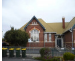
Ascot Vale PS 2608 1885/8 building
