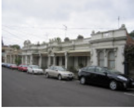
1-11A Shields Street.JPG
