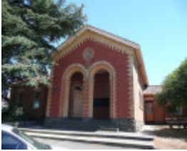
ARARAT COURT HOUSE SOHE 2008
