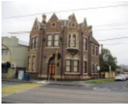
403 - 305 Mt Alexander Road and 1 Bank Street.JPG
