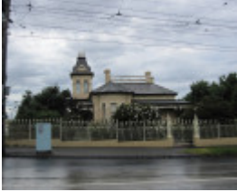
200 Pascoe Vale Road.JPG
