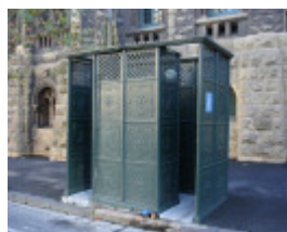
Urinal La Trobe Street exterior KJ 21 06 2007
