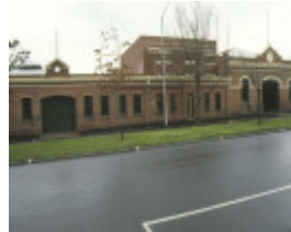
1 former cable tram engine house rathdowne street carlton north street view sep1993
