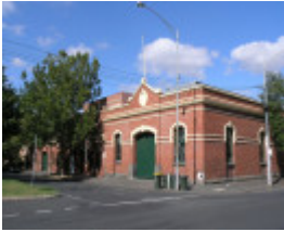
FORMER CABLE TRAM ENGINE HOUSE SOHE 2008
