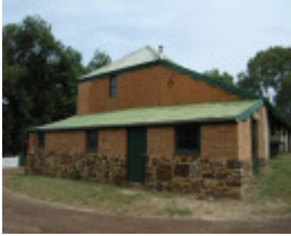
RED BRICK BARN SOHE 2008
