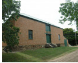
RED BRICK BARN SOHE 2008
