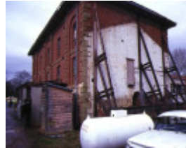
1 flour mill barker street castlemaine front view
