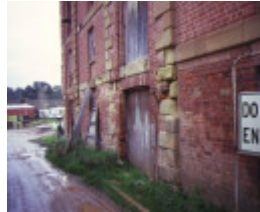
flour mill barker street castlemaine brickwork detail
