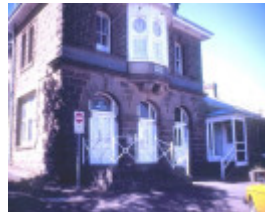
h00618 former ararat post office barkly street ararat front she project 2004
