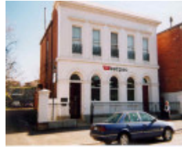
H00131 former bank of nsw barker street castlemaine front elevation
