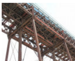
2504_Melton Railway Viaduct_7 November 2009_HV_016_lo res.jpg
