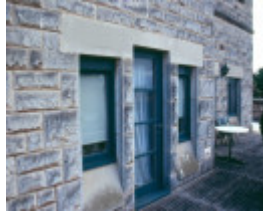
Delgany Portsea 1925 House Windows and Doors September 2003
