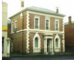
former cbc bank barker street castlemaine corner view
