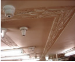
H2100 Myers Melbourne ceiling detail feb2006 jb 047
