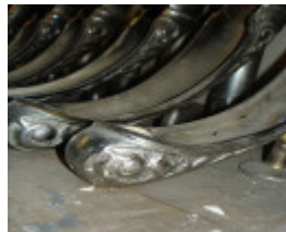
Myers Melbourne Lamson Tubes Detail February 2006
