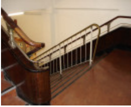
H2100 myers melbourne deco stairs 21 02 06 JB
