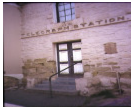
former telegraph office & faulder watson hall barker street castlemaine front view telegraph office
