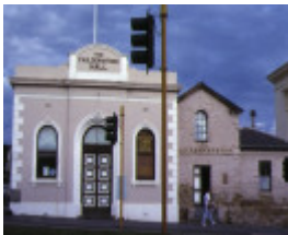
former telegraph office & faulder watson hall barker street castlemaine front view faulder watson hall
