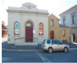
FORMER TELEGRAPH OFFICE AND FAULDER WATSON HALL SOHE 2008
