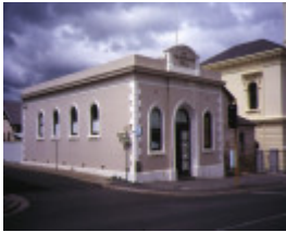
1 former telegraph office & faulder watson hall barker street castlemaine side view faulder watson hall
