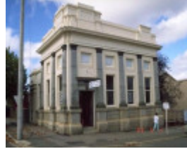
h00580 former state savings bank h0580
