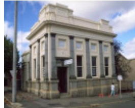
h00580 former state savings bank h0580
