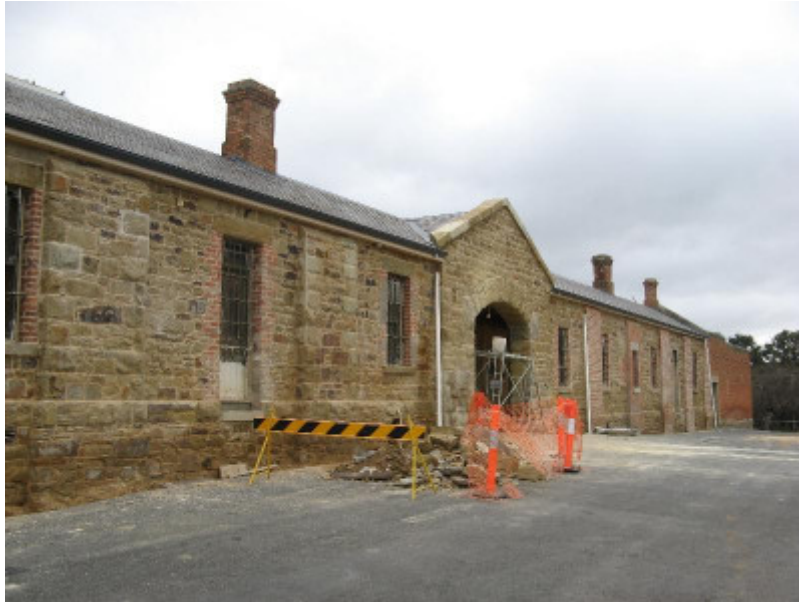
facade conservation as at 25May2011 005.jpg
