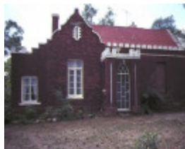
residence farnsworth street castlemaine side view may1984
