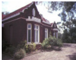
1 residence farnsworth street castlemaine front view may1984
