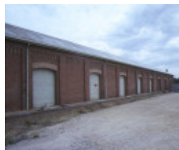
castlemaine railway station complex kennedy street castlemaine railshed side view
