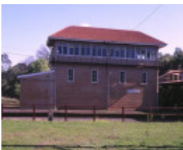
castlemaine railway station complex kennedy street castlemaine signal box
