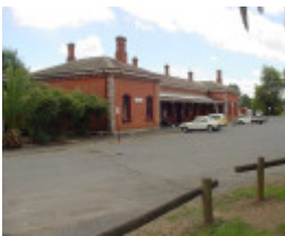
Castlemaine Railway Station View of South East End
