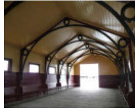
QUEENSLIFF PIER AND LIFEBOAT COMPLEX SOHE 2008
