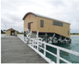
QUEENSLIFF PIER AND LIFEBOAT COMPLEX SOHE 2008
