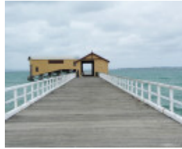
QUEENSLIFF PIER AND LIFEBOAT COMPLEX SOHE 2008
