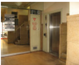
Yule House_lift lobby ground floor_KJ_Oct 09
