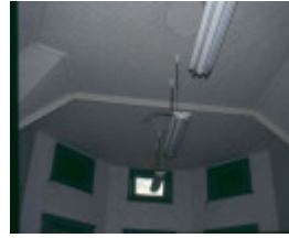
Royal Park Hospital Ward Ceiling April 2002
