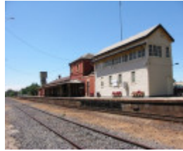
Wangaratta RWS Signal Box & Station Building February 2002
