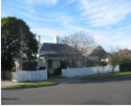
192 Wood Street, Preston
