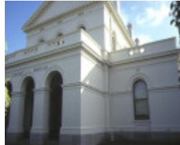
castlemaine court house lyttleton street castlemaine entrance detail aug1984
