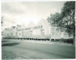
26678 Permewan Wright Sheds
