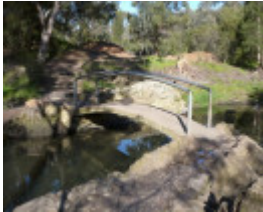
Clifton Bridge, Darebin Parklands (off Separation Street)
