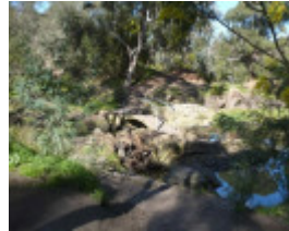
Clifton Bridge, Darebin Parklands, off Separation Street
