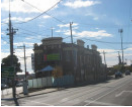
Junction Hotel, 2 - 4 High Street, Preston
