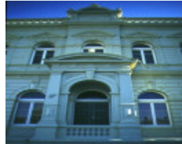
1 former school of mines lyttleton street castlemaine entrance
