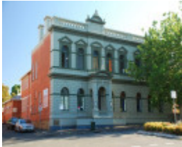
FORMER SCHOOL OF MINES
