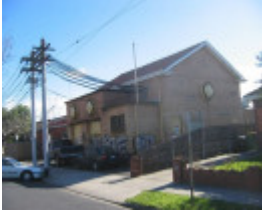
MMTB Substation, 7 Martin Street, Thornbury
