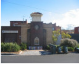
Electricity Substation, Pender Street, Thornbury
