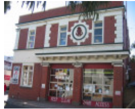
378 High St - Metropolitan Fire Brigade
