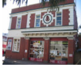
378 High St - Metropolitan Fire Brigade
