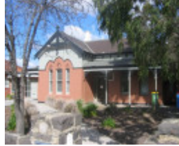
All Saints Anglican Church Complex: Vicarage, 400 High Street
