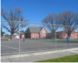
Preston South Primary School No. 824
