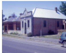
chewton town hall pyrenees highway chewton town hall and post office she project 2003
