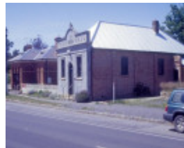
chewton town hall pyrenees highway chewton town hall and post office she project 2003
