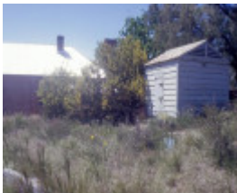
chewton town hall pyrenees highway chewton portable police lock up she project 2003
