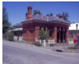
Former Chewton Post Office Pyrenees Hwy Chewton Front and East Wall SHE Project 2004
