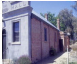
chewton town hall pyrenees highway chewton west wall she project 2003
