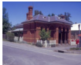
Former Chewton Post Office Pyrenees Hwy Chewton Front and East Wall SHE Project 2004
