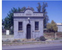
h01015 1 chewton town hall pyrenees highway chewton front she project 2003
