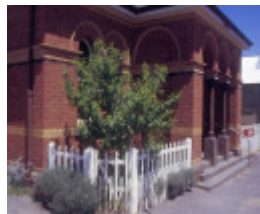
Former Chewton Post Office Pyrenees Hwy Chewton North East Corner SHE Project 2004
