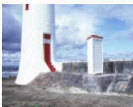
griffith island lighthouse griffith island port fairy entrance
