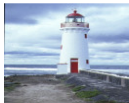
1 griffith island lighthouse griffith island port fairy front view
